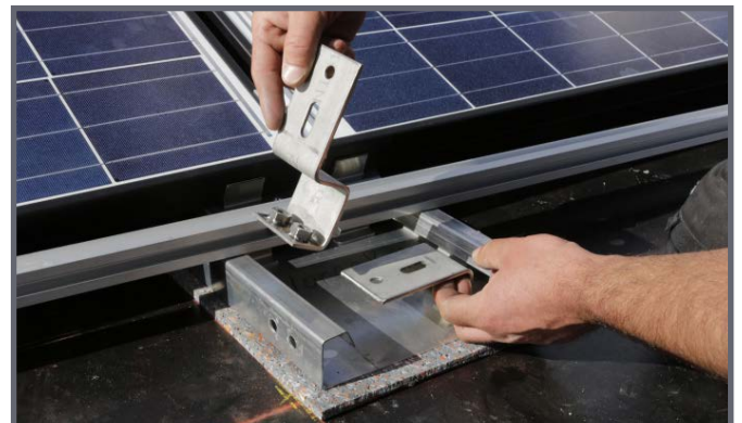
Put the first anchor point into the floor rail
