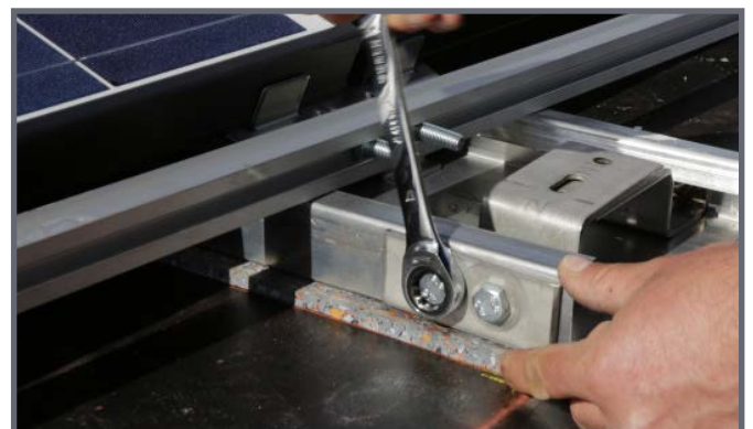
Attach the load distribution plate and screw in the screws!
