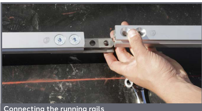
Connecting the running rails
