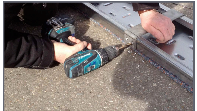
Drill holes in floor rails with drilling template
