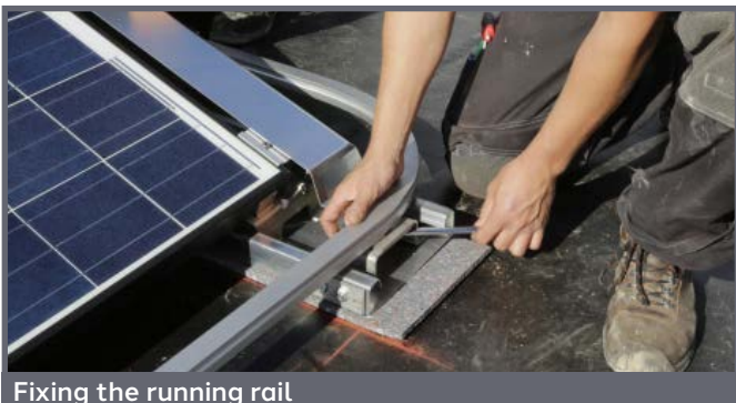
Fixing the running rail
