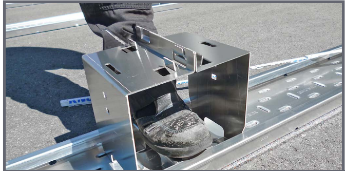
Clicking in the module supports
