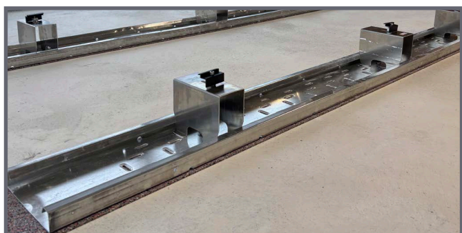
Fully assembled module supports for the first row of modules
