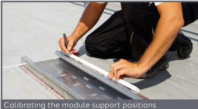
Calibrating the module support positions
