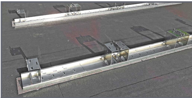
Fully assembled module supports for the first row of modules
