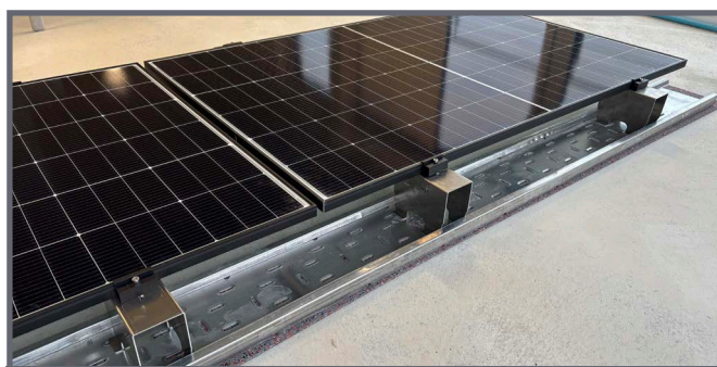
Fully assembled first row of modules
