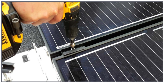
Inserting the module center clamp into the module supports
