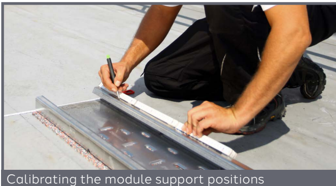
Calibrating the module support positions
